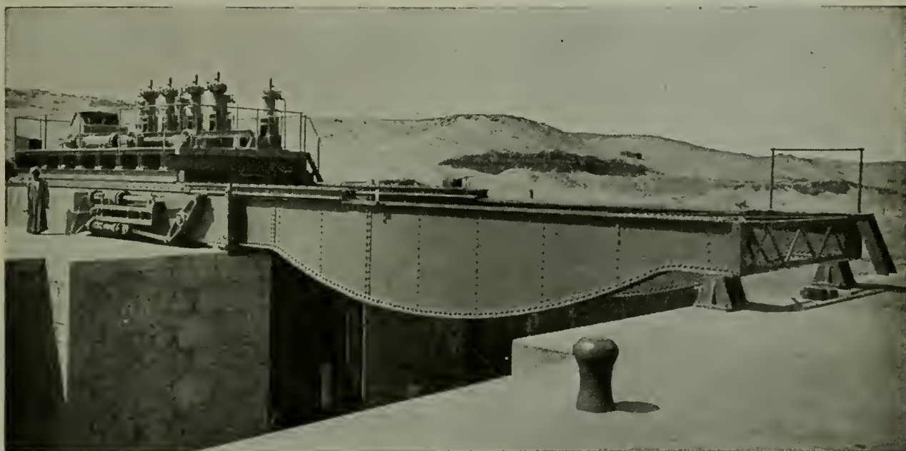
The stored-up waters are released as required through great openings in the dam, and the doors of the openings are so massive that enormous machinery is required to open and close each one.
